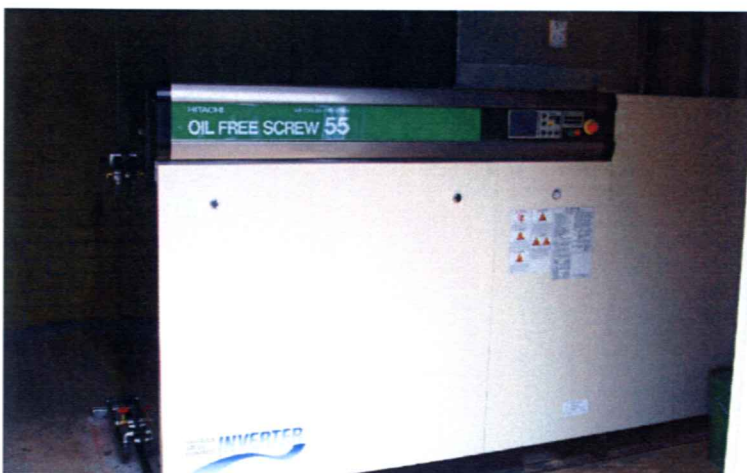
Oil free screw compressor " DSP-55VA61 " at Sara Lee
